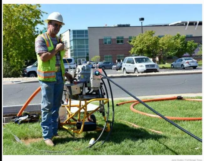
Randy Olson, fiber blowing machine operator from Schumann Communications, oversees the pulling of fiber optic cable through the conduits under Riverview Avenue
